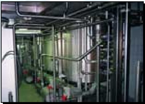
Leveltransmitters on CIP tanks
