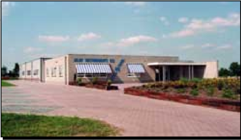
Factory Klay Instruments B.V. at Dwingeloo, The Netherlands
